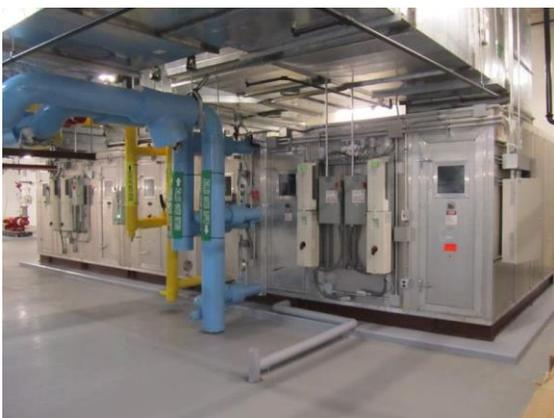
Fig. 1 24,000 CFM VAV Air Handling Unit with 48"H x 60"W main supply duct. Unit is 20'L x 8'W x 7'H
