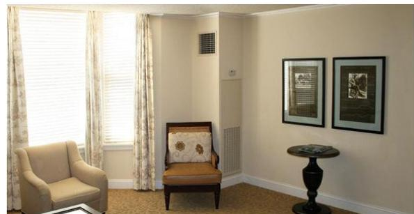
Fig. 2 Typical fan coil furred in with supply and return grill
