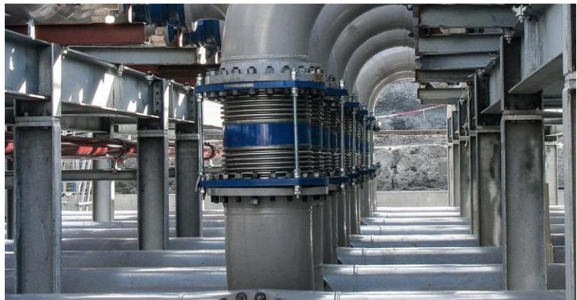
Fig 2.0 In-Line Rubber or Stainless Steel Thermal Expansion Compensators
