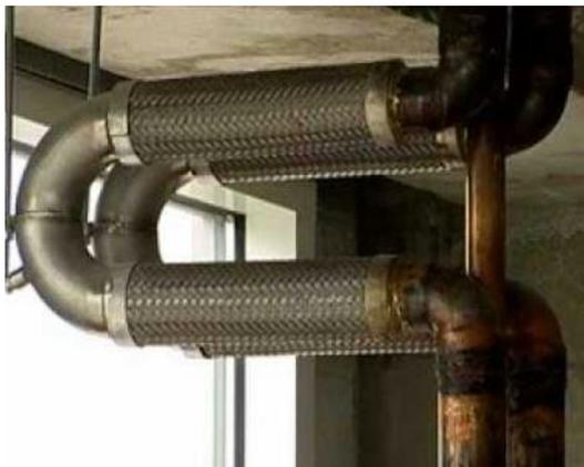
Fig. 1.0 Horizontal Thermal Expansion Loops
