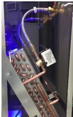
Position of the stub-out in the cabinet riser slot
