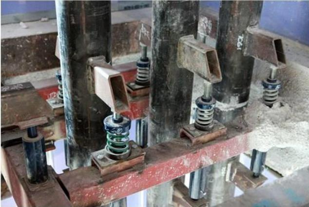
Fig. 3.0 Full Floating Riser System using Spring Isolators
