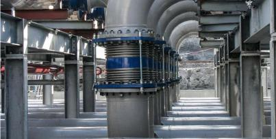
Fig. 1.0 Horizontal Thermal Expansion Loops
