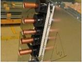
installation time is reduced by 30 minutes per unit by having to solder only one joint
