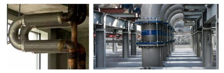
Fig. 1.0 Horizontal Thermal Expansion Loops
