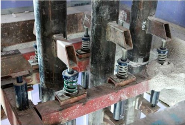
Fig. 7 Full Floating Riser using Spring Isolation
