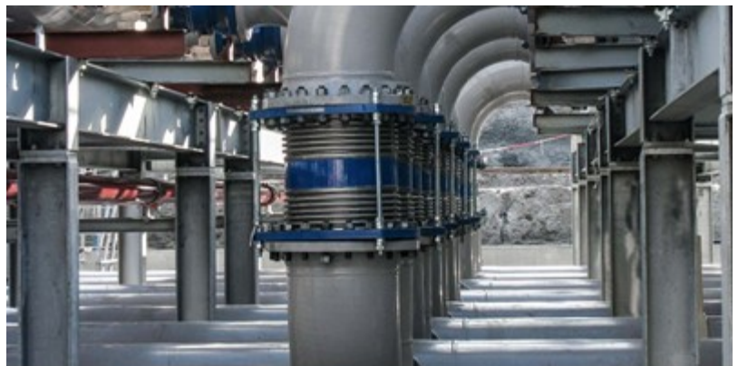
Fig. 6 In-line Rubber or Stainless Steel Thermal expansion compensators
